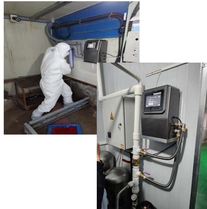
*Installing a Silver Ion Generator
