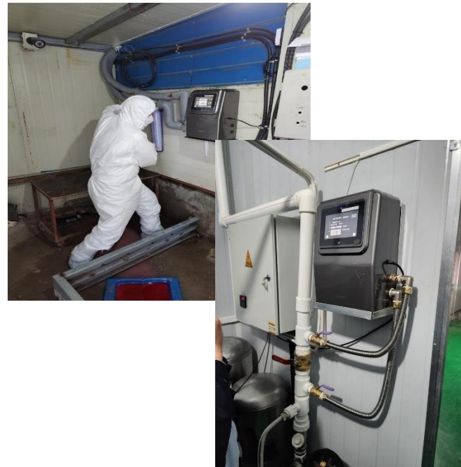
*Installing a Silver Ion Generator
