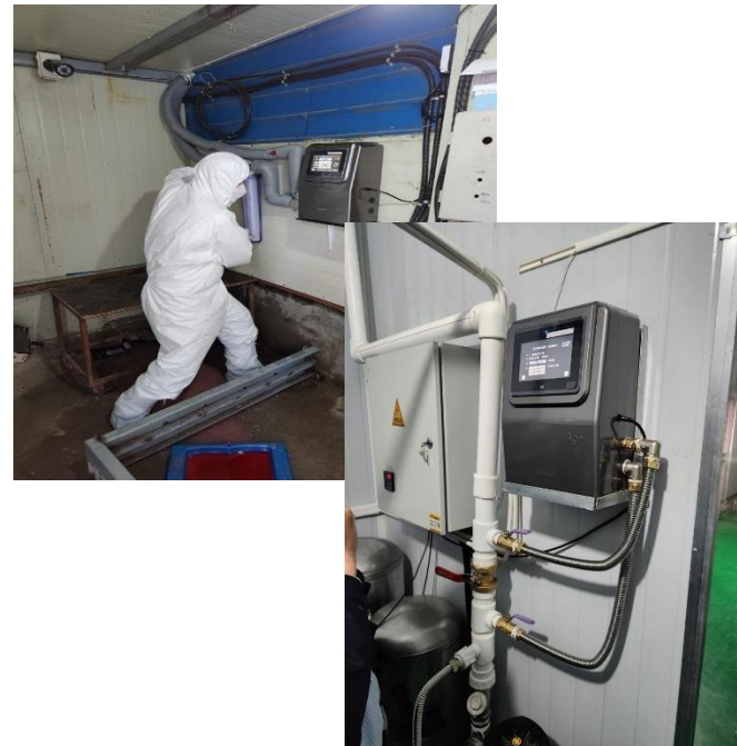
*Installing a Silver Ion Generator
