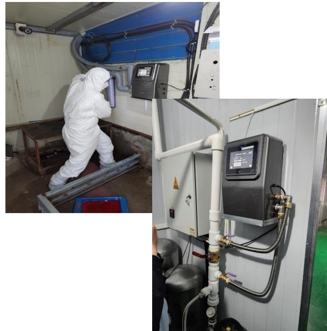
*Installing a Silver Ion Generator
