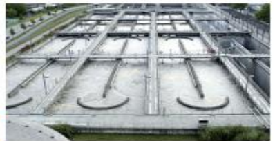
Wastewater, Sewage Treatment
