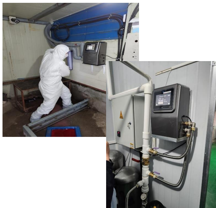
*Installing a silver ion generator
